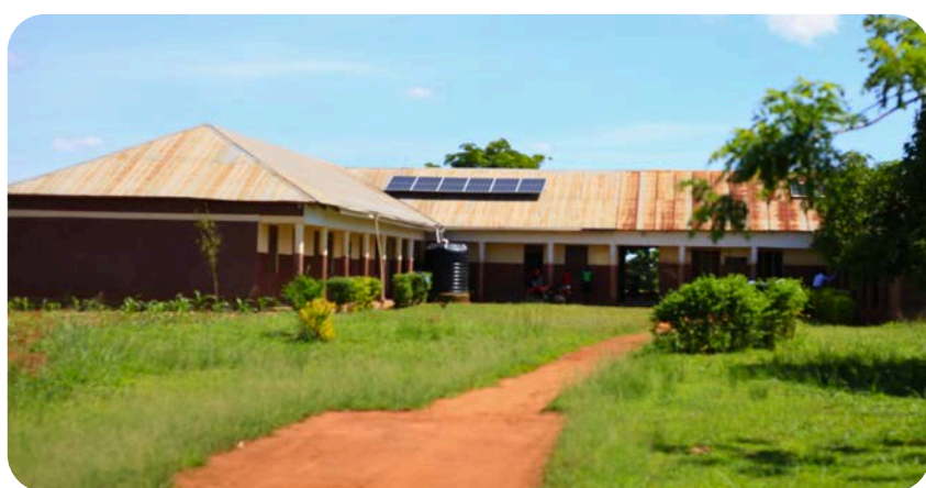
The formation house needing renovation
