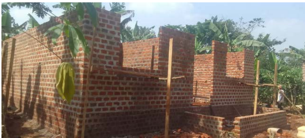
Progress being made on the family's new home
